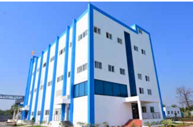
KILO LAB (SCALE UP FACILITY), PANCHDEVLA
