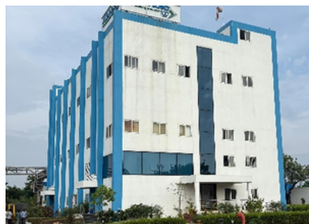
KILO LAB (SCALE UP FACILITY)
