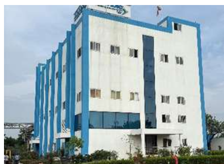
KILO LAB (SCALE UP FACILITY)
