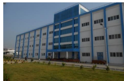
API Plant-3 at Karkhadi, Gujarat
